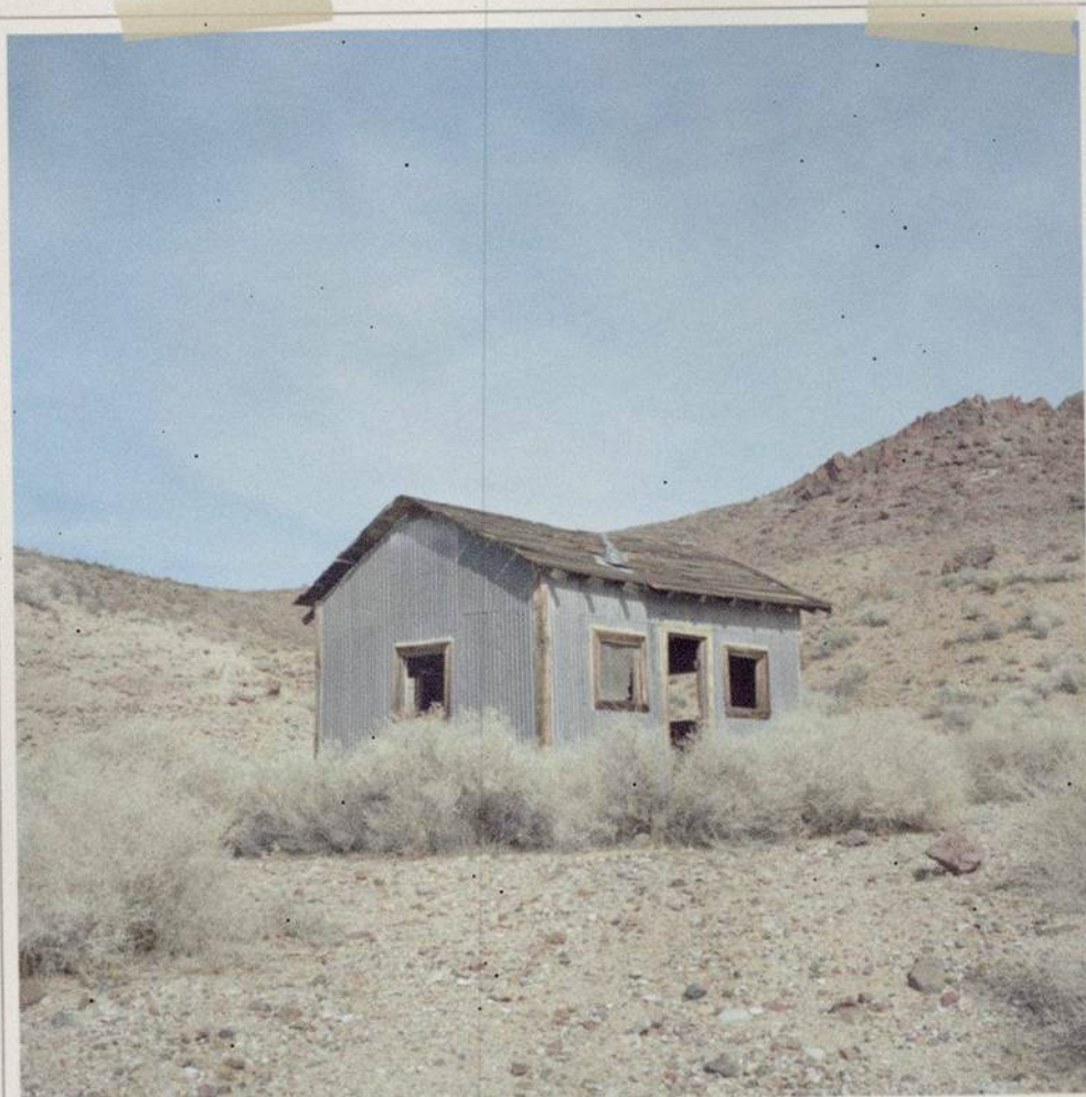
PHOTO 1 OUTBUILDING, FROM THE ACCESS TRACK, LOOKING NORTH
