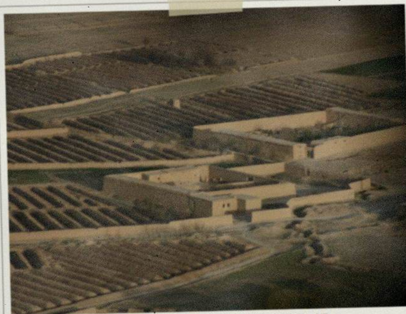
PHOTO 3 COMPOUND FROM THE RIDGE, LOOKING EAST
